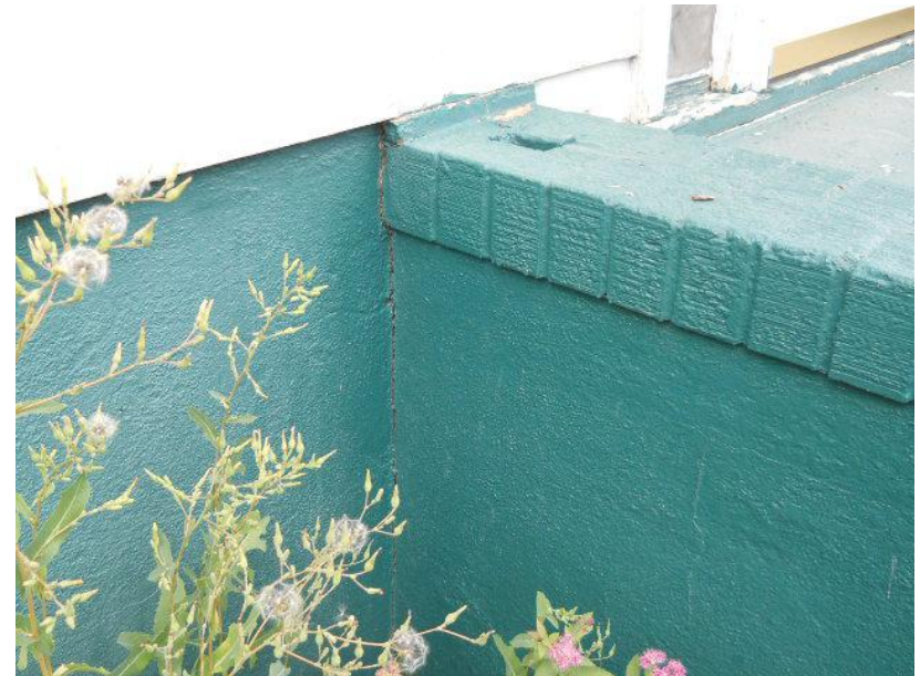
8/25/2011 12:32:24 PM View Northwest of South Side of Front Stairs - Note Open Crack Between the Stairs and Foundation 501 Broadway Avenue South, Red Lodge, MT 2011-08-25 12-32-24 - 0096.JPG
