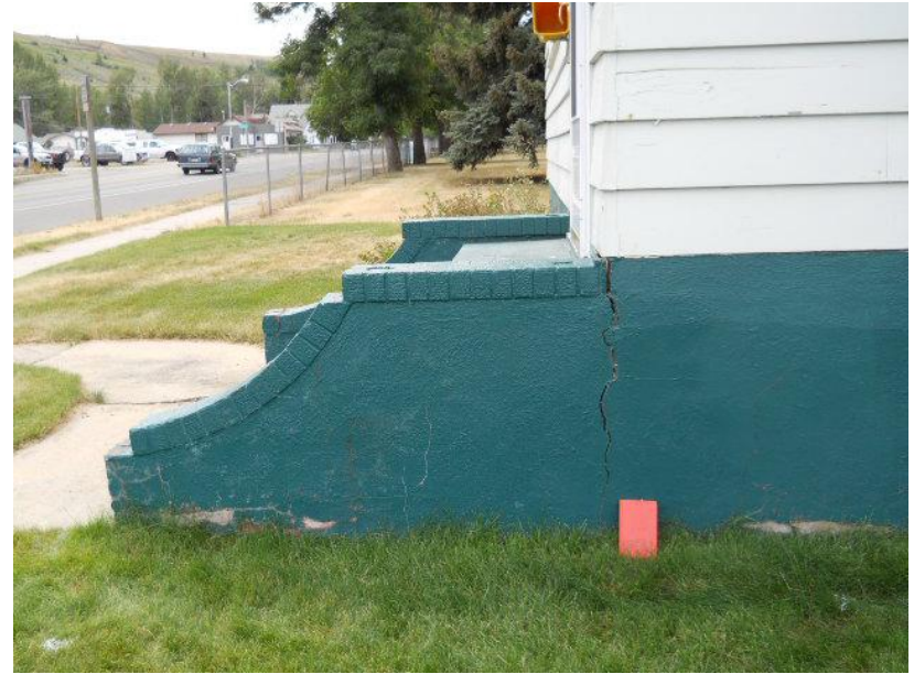
View South of Front Stairs - Note Open Crack Between the Stairs and Foundation 501 Broadway Avenue South, Red Lodge, MT 2011-08-25 12-33-47 - 0098.JPG
