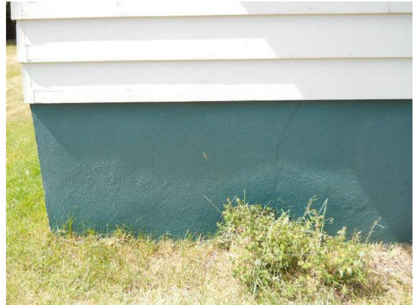
View West of East Foundation and Hairline Crack 1 near Southeast Corner of House 501 Broadway Avenue South, Red Lodge, MT 2011-08-25 12-57-55 - 0100.JPG
