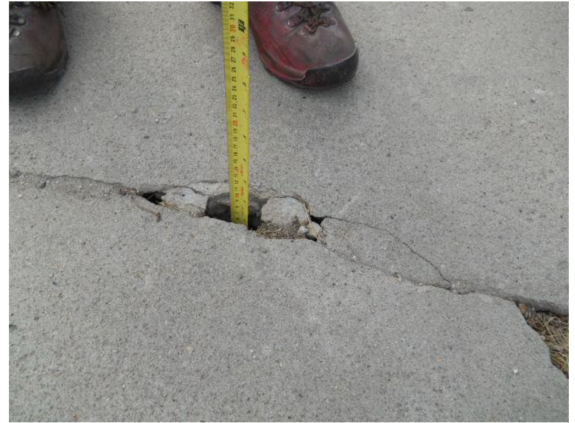
8/25/2011 12:30:32 PM View South of Sidewalk - Crack is Open to a Depth of 4 Inches 501 Broadway Avenue South, Red Lodge, MT 2011-08-25 12-30-32 - 0090.JPG
