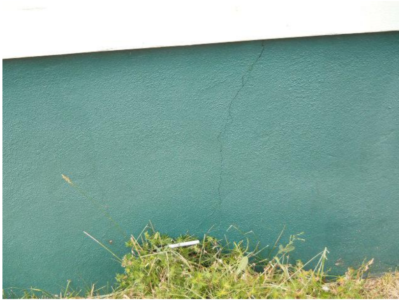
View West of East Foundation and Hairline Crack 1 near Southeast Corner of House 501 Broadway Avenue South, Red Lodge, MT 2011-08-25 12-58-39 - 0101.JPG
