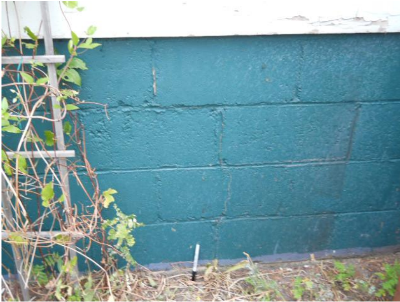
8/25/2011 1:01:16 PM View East of West Foundation and Crack 5 in CMU Block 501 Broadway Avenue South, Red Lodge, MT 2011-08-25 13-01-16 - 0105.JPG
