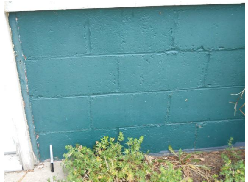
8/25/2011 1:01:41 PM View East of West Foundation and Paint Peeling or Possible Cracking in CMU Block 501 Broadway Avenue South, Red Lodge, MT 2011-08-25 13-01-41 - 0106.JPG
