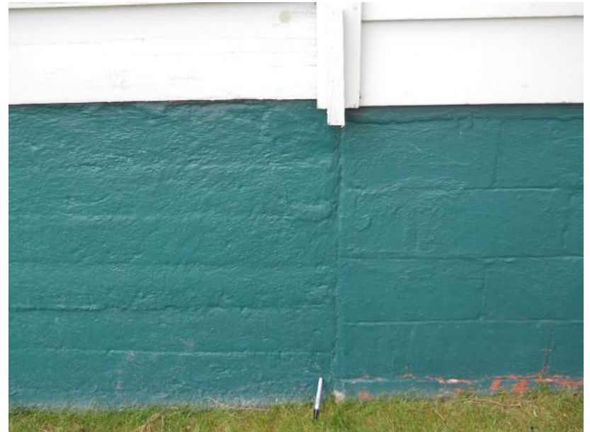
8/25/2011 1:03:05 PM View South of North Foundation and Hairline Crack 6 at Back Addition 501 Broadway Avenue South, Red Lodge, MT 2011-08-25 13-03-05 - 0108.JPG
