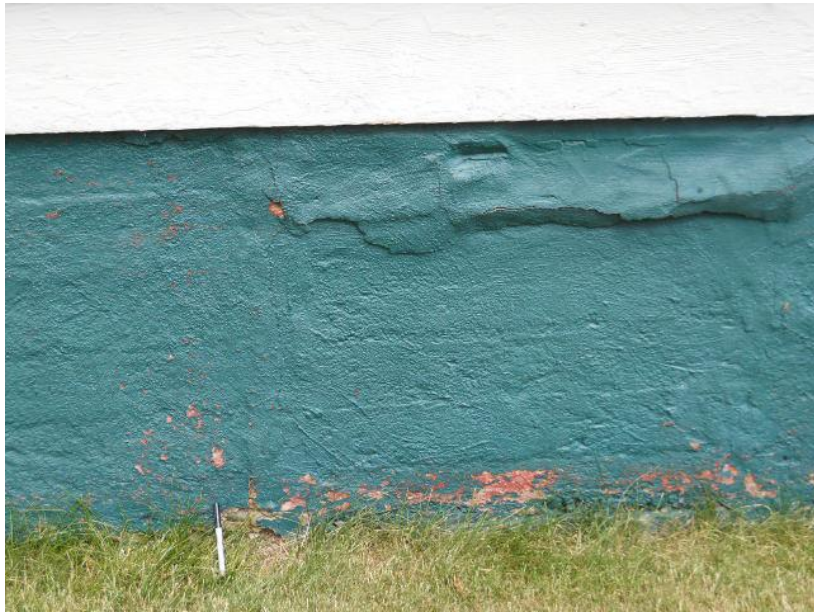
View North of South Foundation and Buckled Stucco and Hairline Crack 3 501 Broadway Avenue South, Red Lodge, MT 2011-08-25 13-00-21 - 0103.JPG
