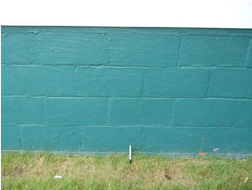
8/25/2011 1:02:54 PM View South of North Foundation and Paint Peeling or Possible Cracking in CMU Block 501 Broadway Avenue South, Red Lodge, MT 2011-08-25 13-02-54 - 0107.JPG
