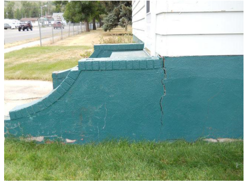
8/25/2011 12:31:35 PM View South of Front Stairs - Note Open Crack Between the Stairs and Foundation 501 Broadway Avenue South, Red Lodge, MT 2011-08-25 12-31-35 - 0094.JPG
