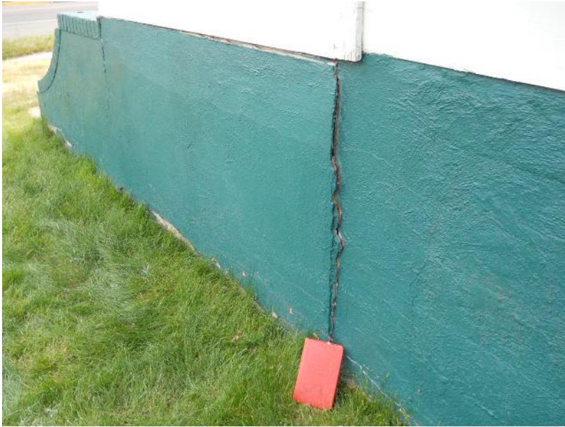
View Southeast of North Foundation and Open Crack 7 in Stucco Where the Front Addition and Main House Foundation Meet 501 Broadway Avenue South, Red Lodge, MT
